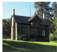
Fort Dalles Surgeon's Quarters
