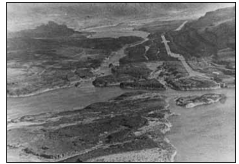
The Celilo canal (right) was cut through the basalt rock to bypass the treacherous narrows of the "dalles" rapids (to the left).
