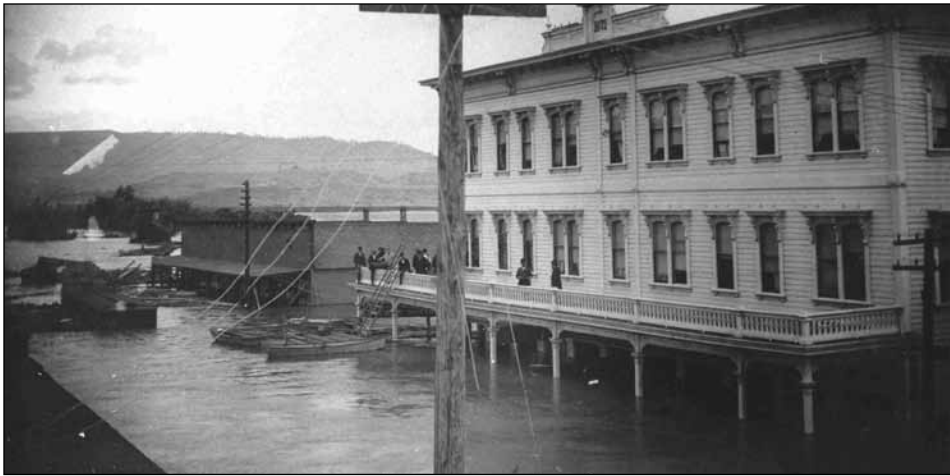
The Umatilla House during the flood of 1894. The photo, taken atop a railroad car, looks west. Photo courtesy of Fort Dalles Museum, #D2588
