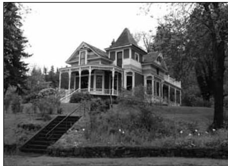
Jefferson Mosier House.
