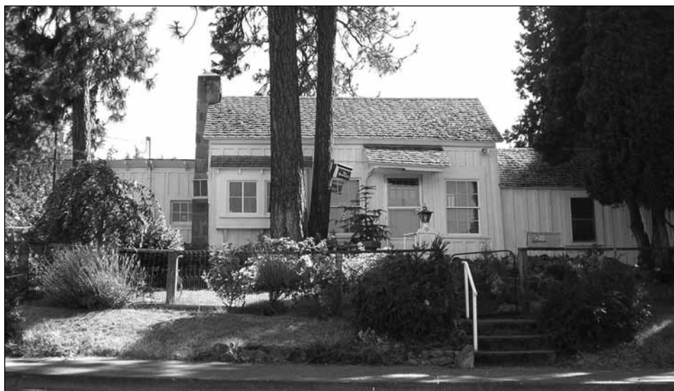
THE RORICK HOUSE is believed to have been built in the early 1850s for a non-commissioned officer at Fort Dalles.
